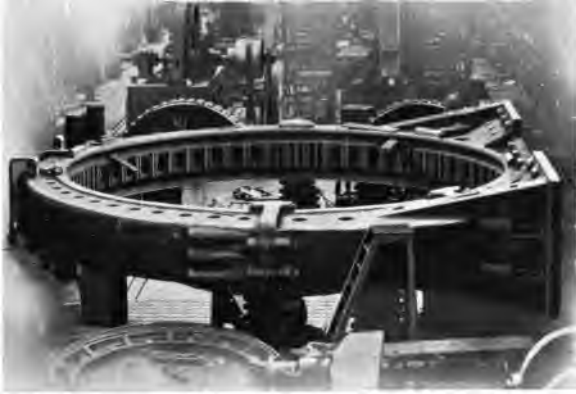
5000 KW Generator in Course of Construction
